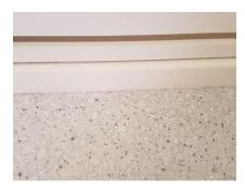
Photo 4 - After vinyl is fitted any excess silicone that squeezes up is removed.
