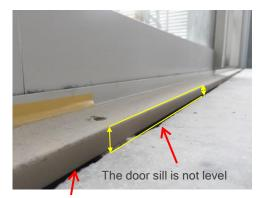
A gap between the concrete and door sill will not allow the vinyl floor covering to finish neatly against it.
